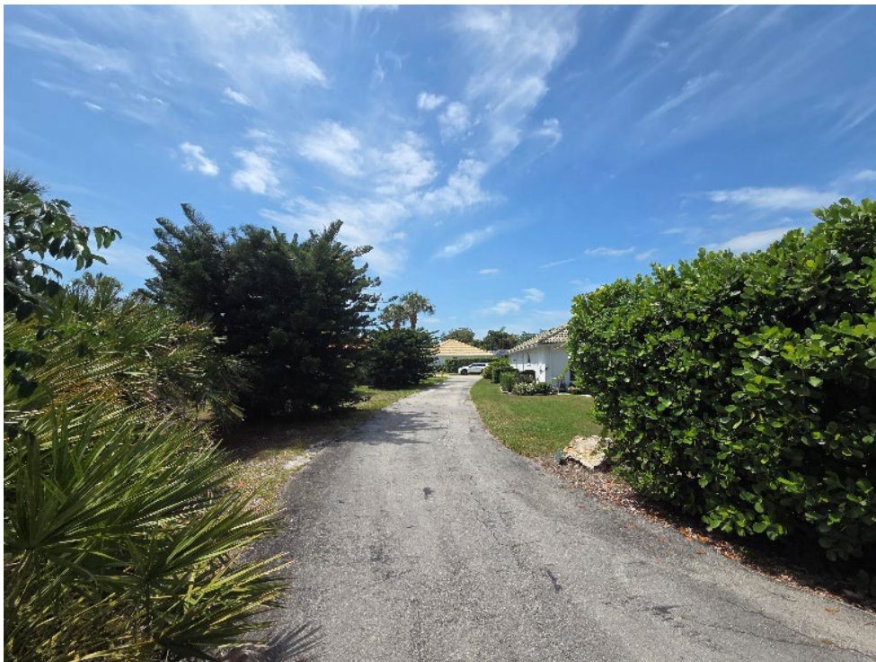
Site Photograph 16 – Looking south along the 20-foot-wide utility easement
