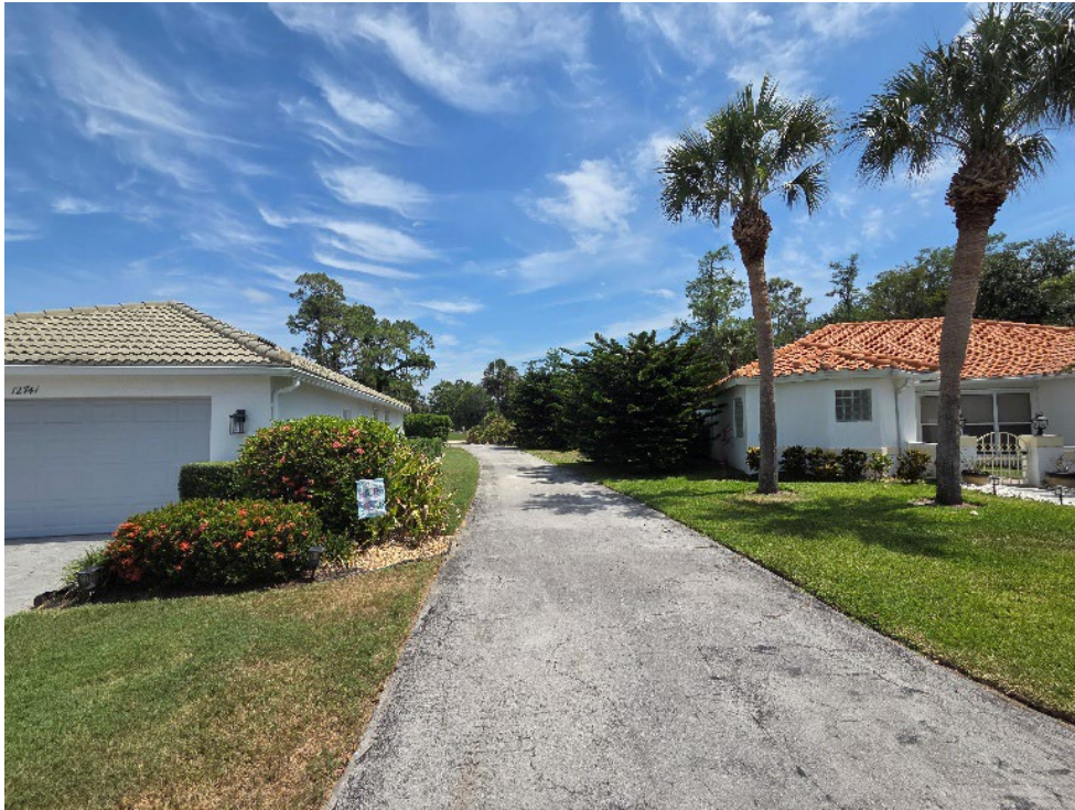
Site Photograph 11 – Looking north along the 20-foot-wide utility easement
