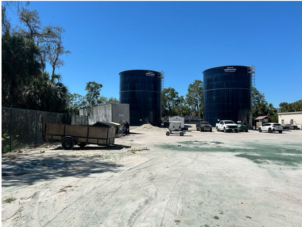
Site Photograph 4 – Looking west at the Site
