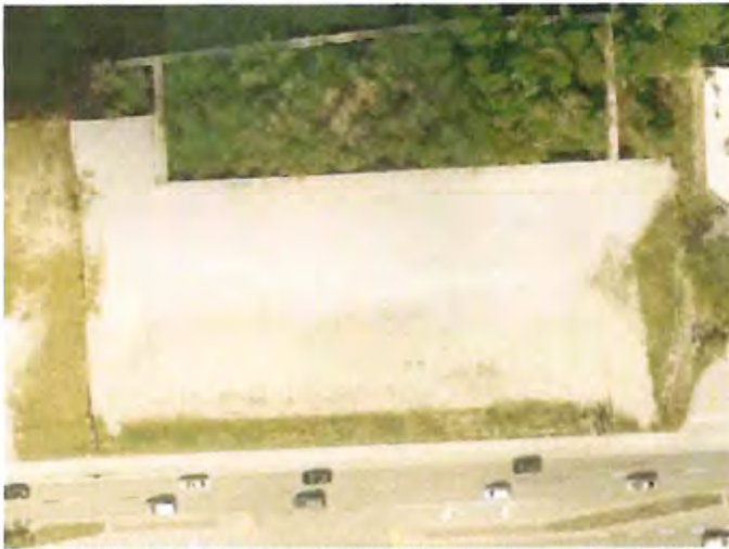
Title: 2011 Aerial Image of 4570 Bonita Beach Road SW
