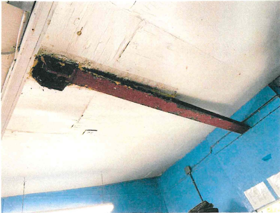
Lead Paint-Pole Barn
