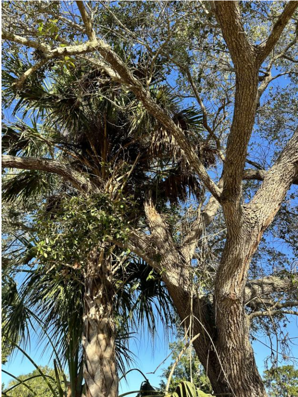
Photo 2: View of Tree #1 showing broken trunk.
