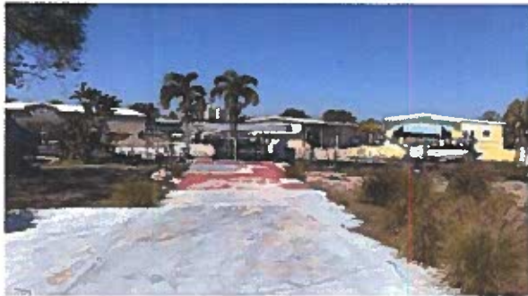
Building Front Photo
