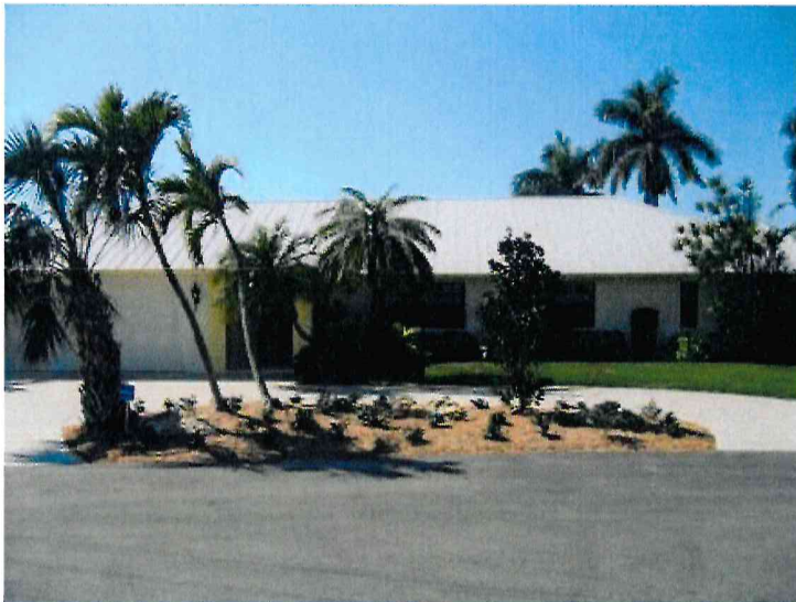
Building Front Photo
