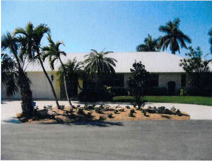
Building Front Photo
