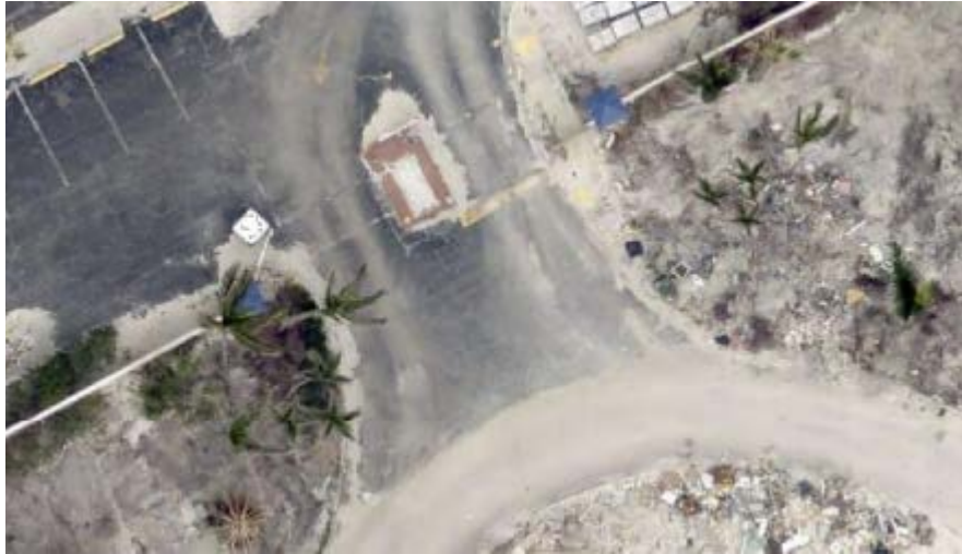
10/2023: Entryway Destroyed by Hurricane Ian
