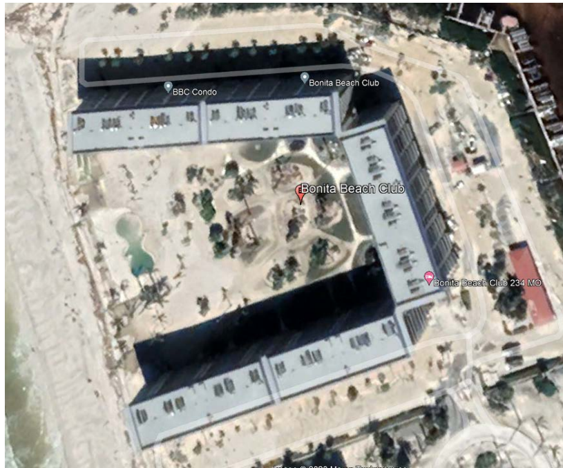
10/2022- Damage by Hurricane Ian
