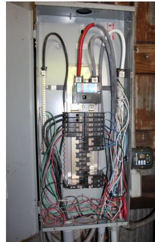
Barn panel, interior
