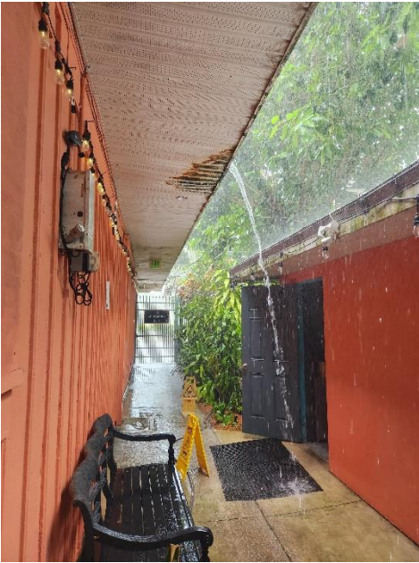
Rainwater off Main Valley at Restrooms
