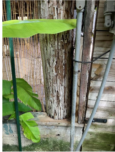
Pole Column – Typical Embedment in Foundation Wall
