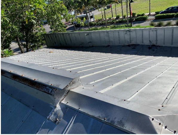
View from Ridge – Storefront Roof Valley
