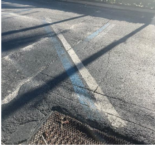
Overlaying parking striping
