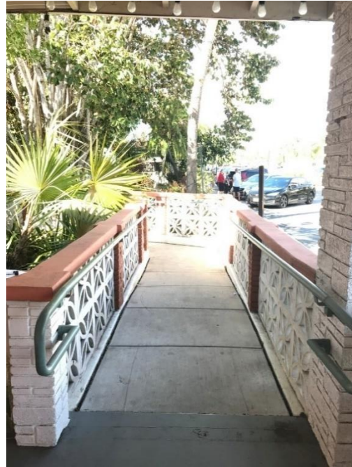
Front entrance ramp and stair photos
