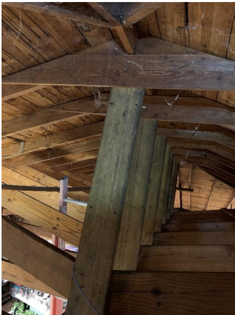
Custom Built Wood Trusses
