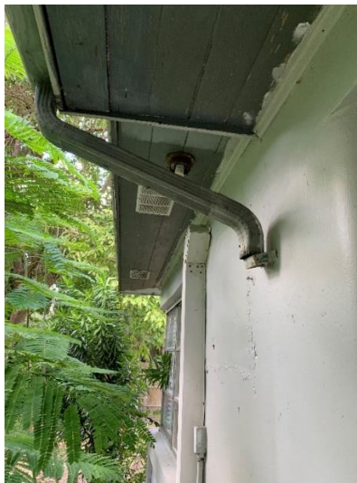
Downspout at Sidewall
