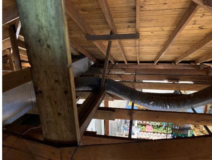
Long Span Rafters with Post to Ceiling
