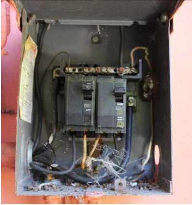
Exterior, 4 circuit load center
