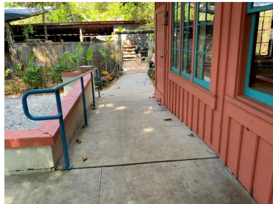
Rear ramp photos
