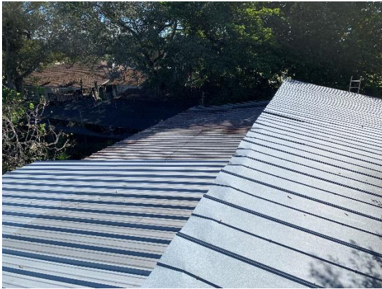
Light Gage Roofing
