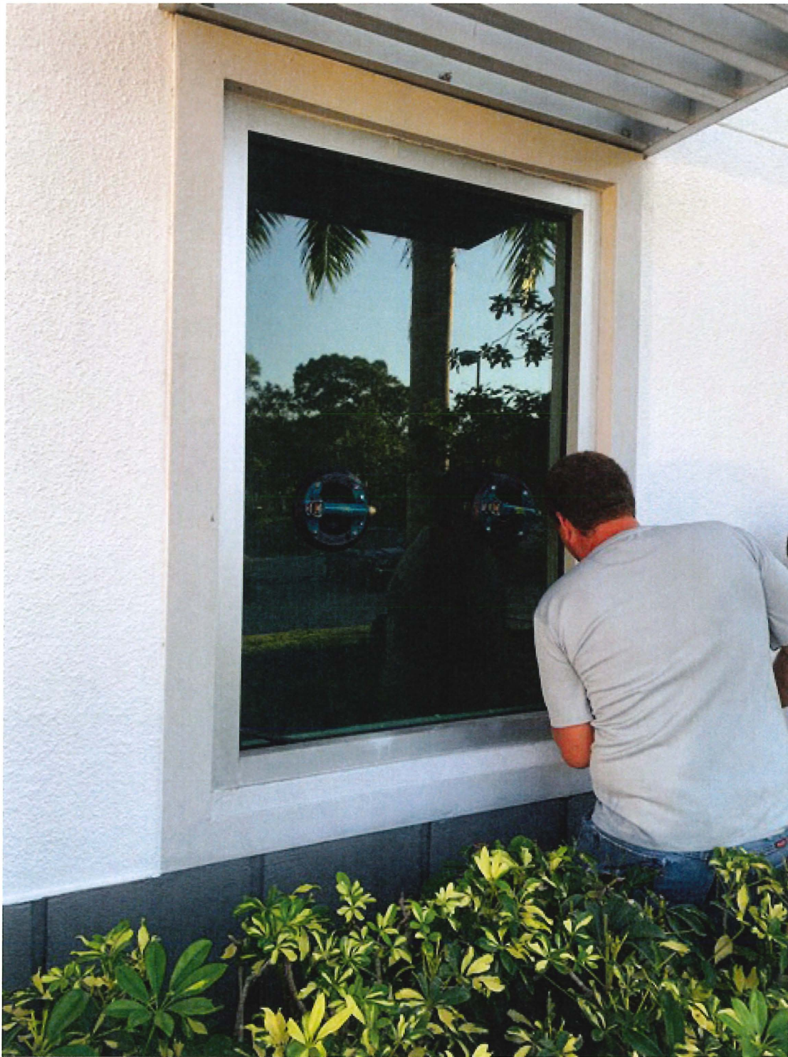
LOCATION OF WINDOW REMOVAL
