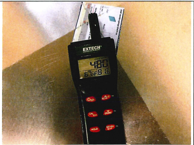
Photo 20: Mechanical Room 116 – Overview of temperature, relative humidity and carbon dioxide readings.
