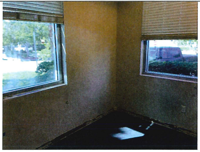
Photo 32: Office 106 - Overview of assessed area.
