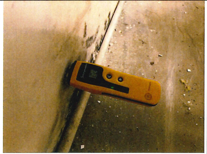
Photo 18: Mechanical Room 116 – Elevated moisture was not detected.
