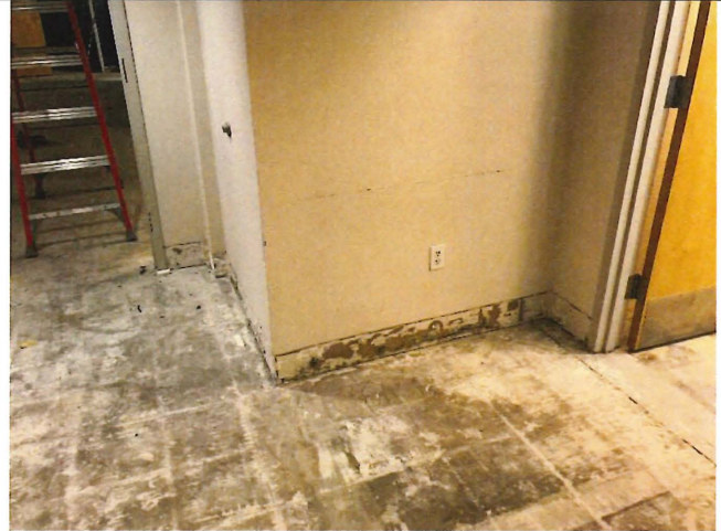
Photo 10: Stair 201A/Vestibule201/Adjacent Cubicles- Overview of assessed area.
