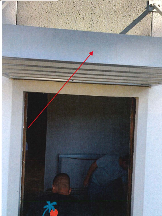
SUNSHADE INSTALLED ABOVE WINDOW OPENING
