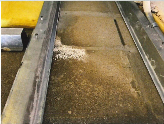
Photo 3: City Manager 220-Efflorescence was observed on the block wall.
