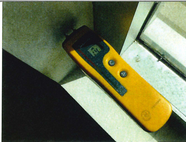
Photo 5: Break Room - Elevated moisture was not detected.
