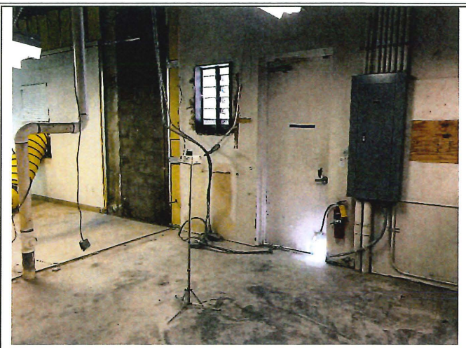
Photo 12: Mechanical Room 116 – Overview of assessed area.
