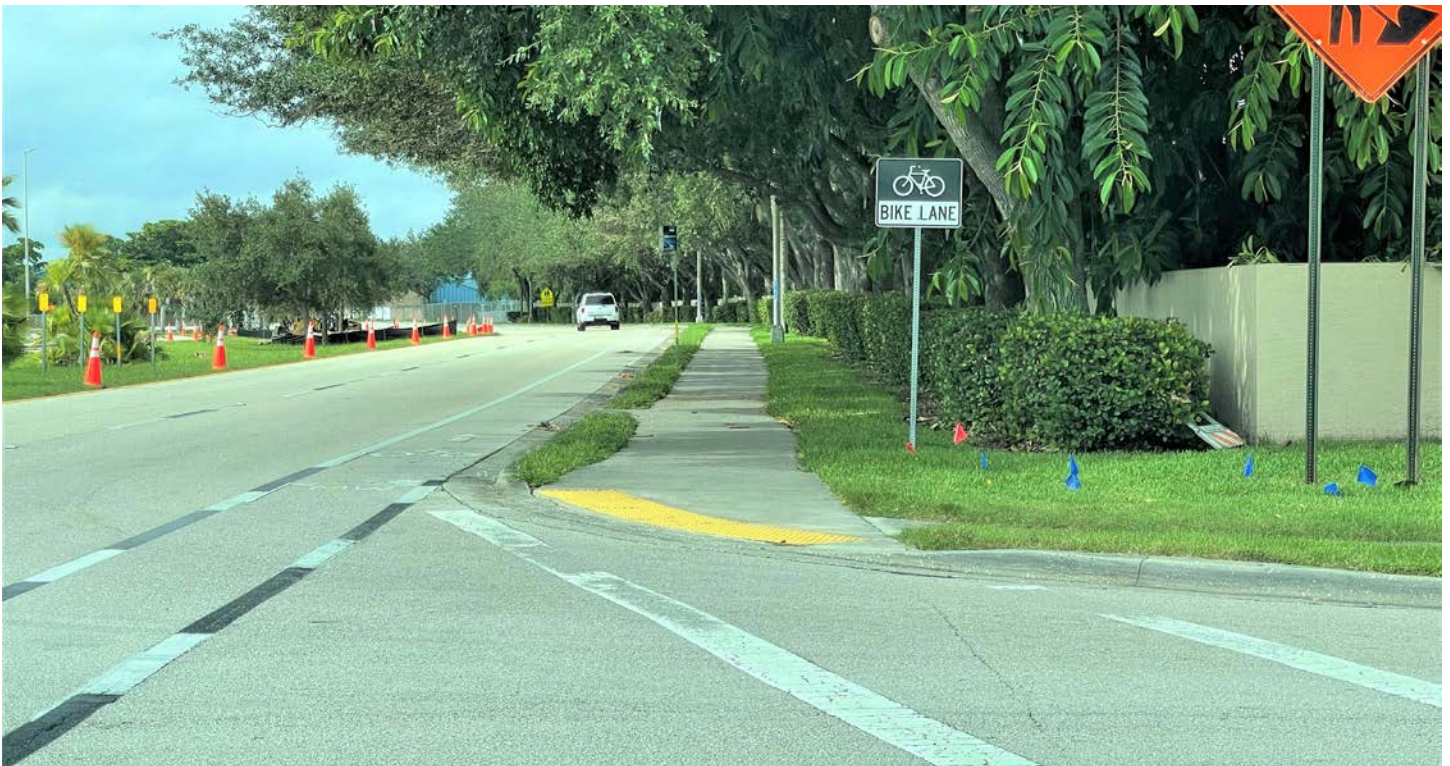
Three Oaks Parkway looking south
