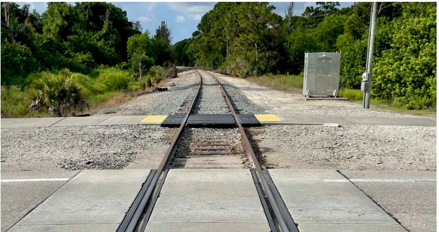
Rail crossing at Corkscrew Road looking north
