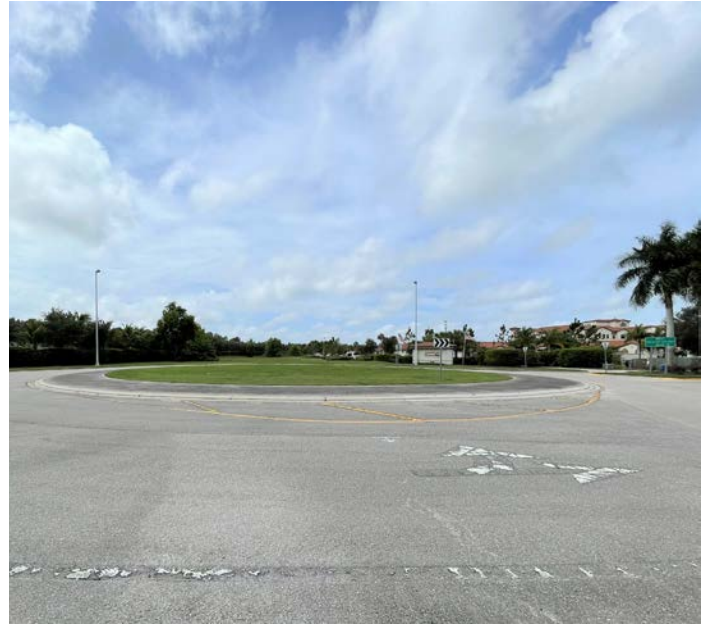
Via Coconut Road roundabout looking south toward Production Boulevard
