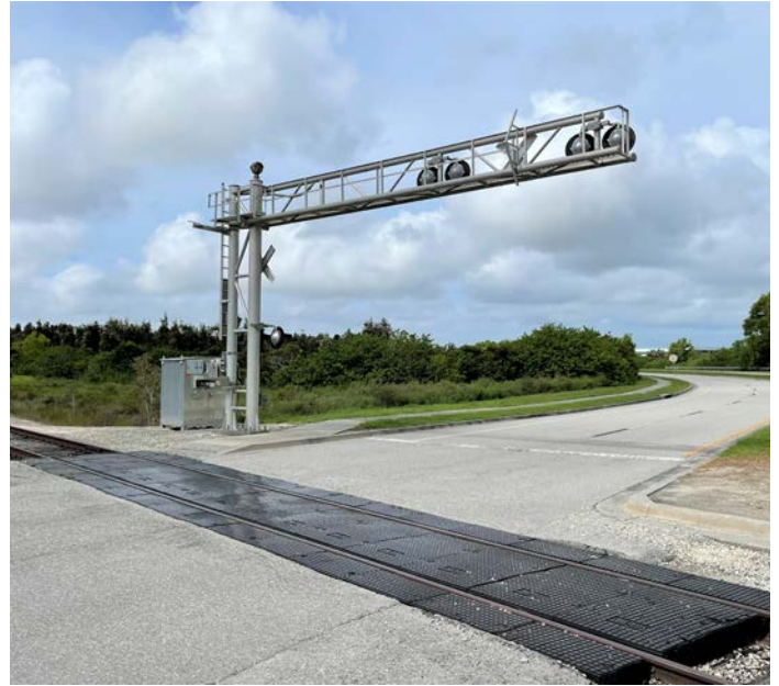
Rail crossing at Coconut Road looking southwest
