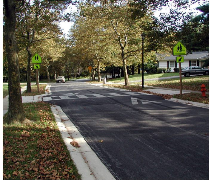
A raised crosswalk in a residential area Pedbikeimages / Dan Burden
