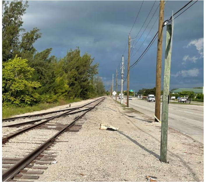
Rail spur on Alico Road looking west
