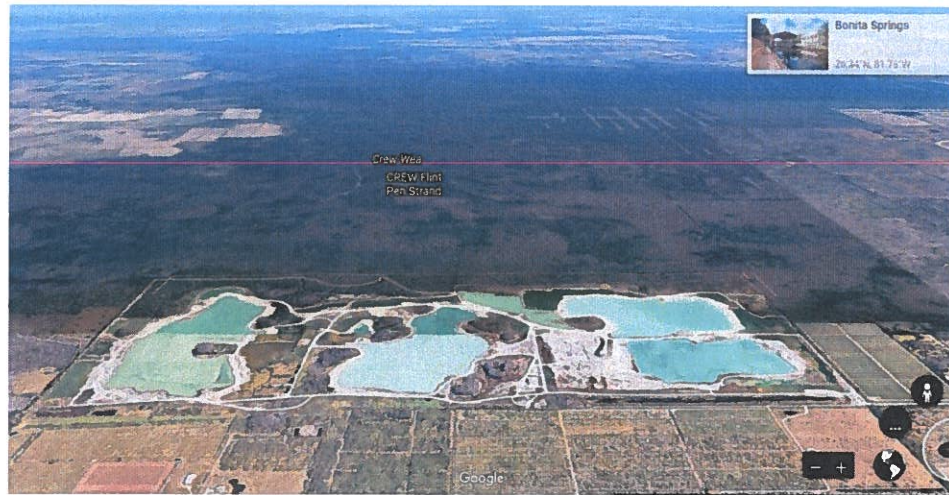
Mine Property and Agricultural Properties View Perspective to the East Source: Google Earth
