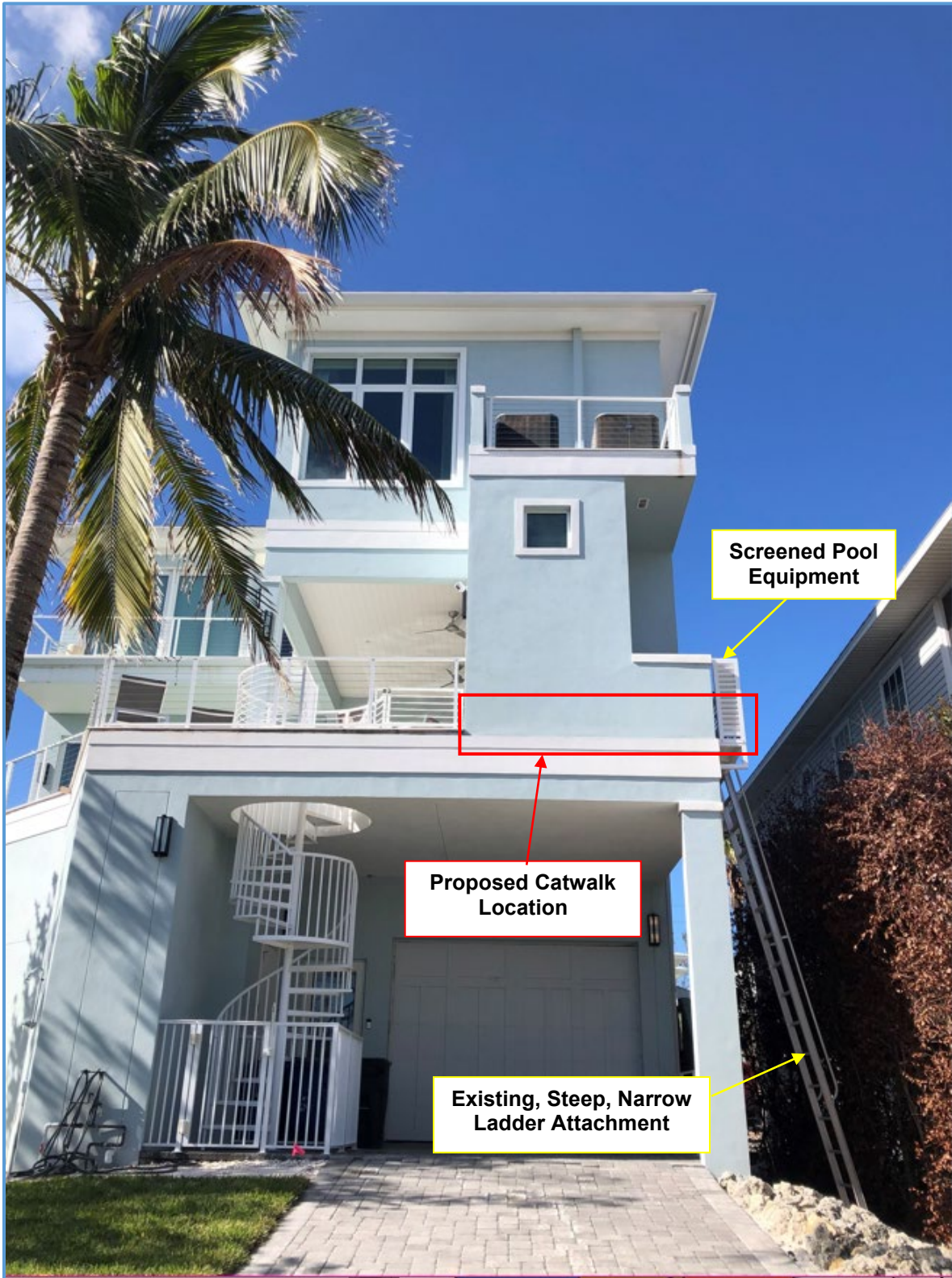
Figure 3 – Existing Conditions – Rear View
