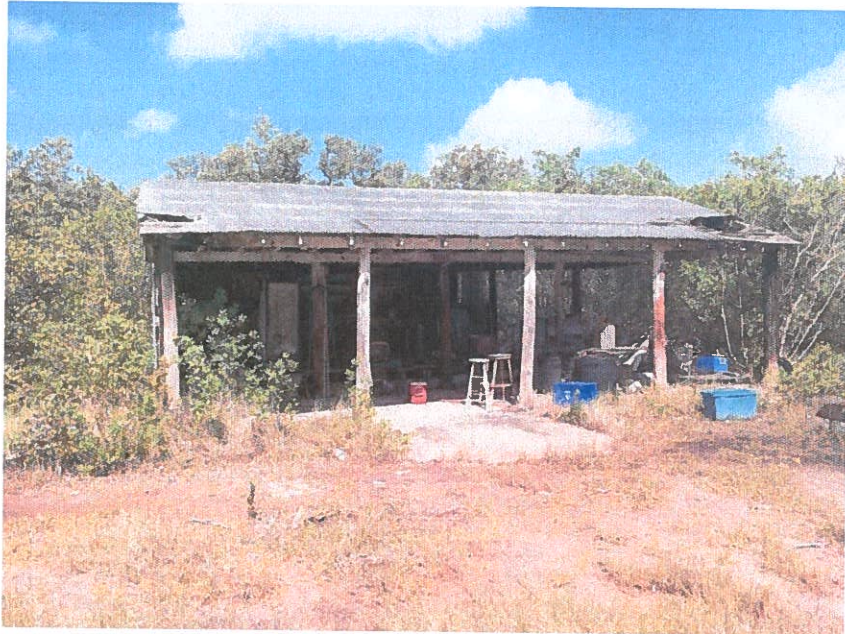
Figure 8. View west of pole barn in northwest corner of parcel.
