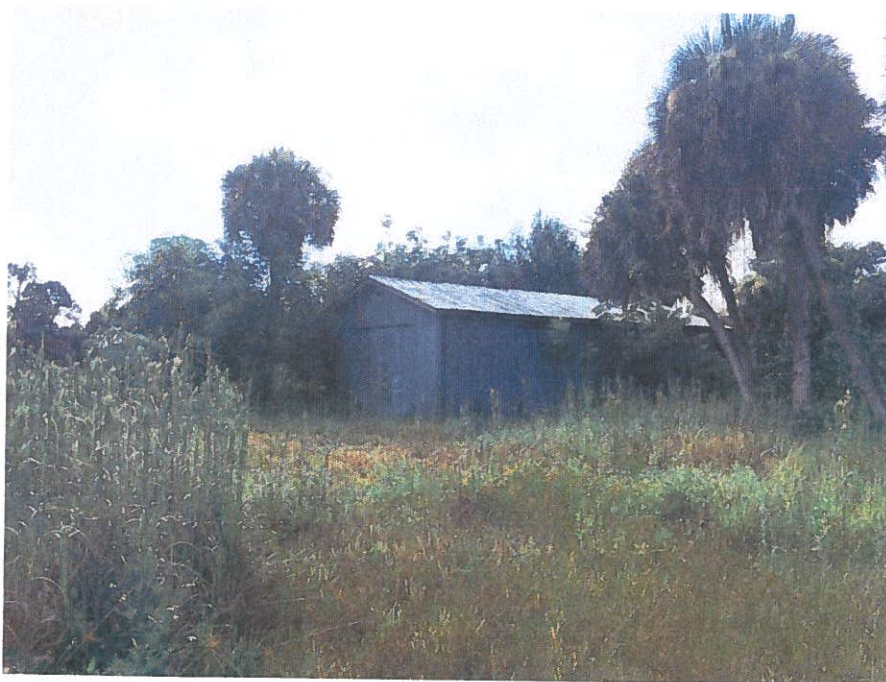
Figure 3. View southeast at the Week' Maintenance Shed building, 8LL2630, a historic structure recorded in 2013.
