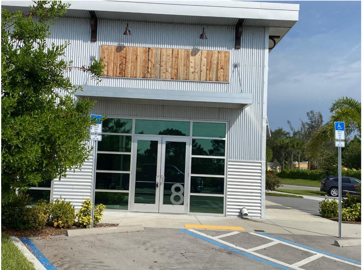
1 Existing pedestrian access doors-M8
