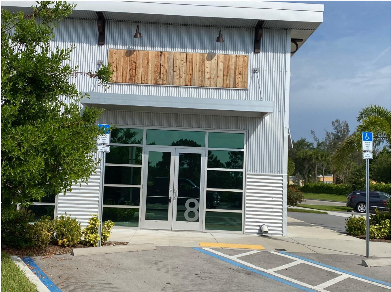
1 Existing pedestrian access doors-M8
