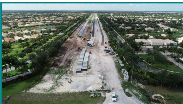
View of Logan Boulevard during construction.
